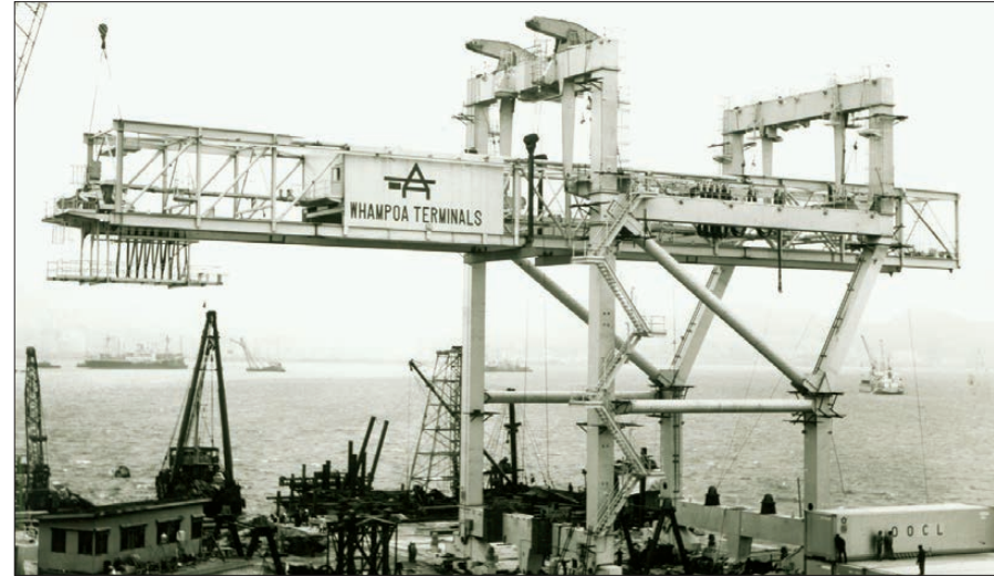
Low-profile Portainer cranes had an outreach limited to five or six containers
