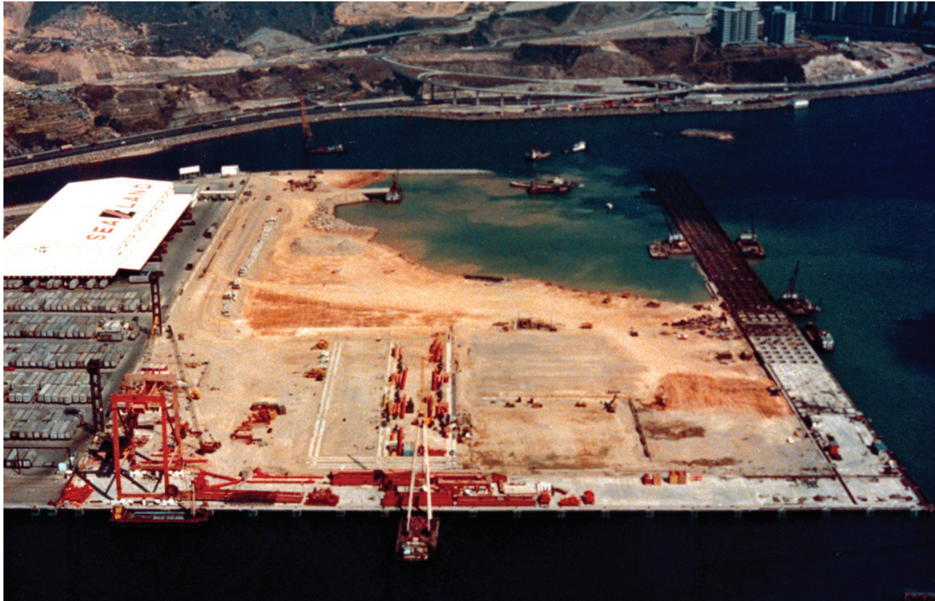
Land reclamation progressed rapidly. Millions of cubic yards of mud were dredged and replaced with sand fill. Terminal 4 was completed in 1976, two years after the land was granted
