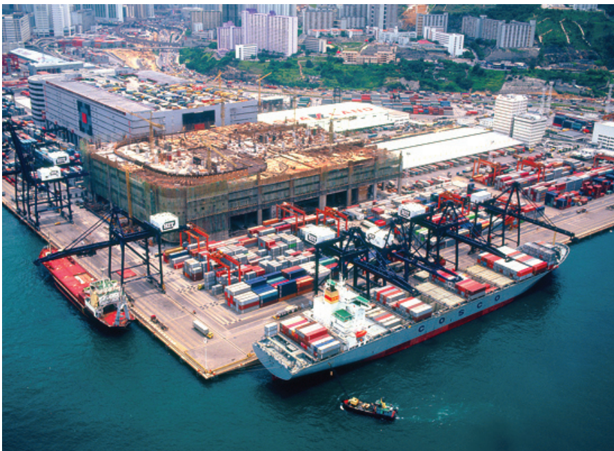
The first phase of the Hutchison Logistics Centre started operations in 1991 while the building was still under construction. The ground floor of the building is used to stack containers as part of the Terminal 4 container yard
