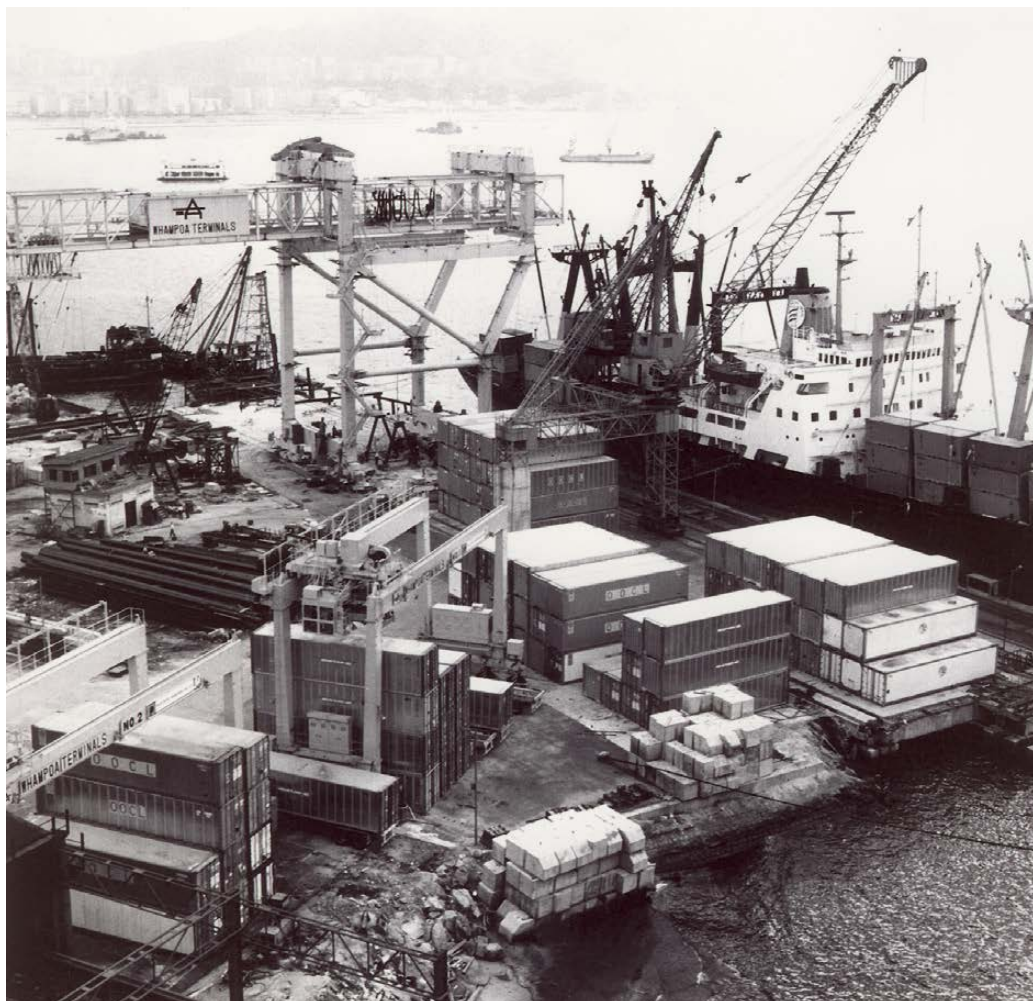
Some berths were redesigned to accommodate containers at Whampoa Terminals. With the introduction of Portainer cranes (top left) and some early rubber-tyred gantry cranes (bottom left), the terminals were able to handle both containers and general cargo
