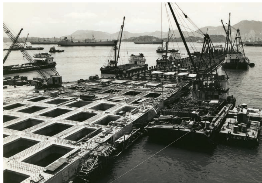
The construction of Terminal 4 involved over 40,000 metres of steel piling, which were driven into place to form an 881-metre-long quay with three berths
