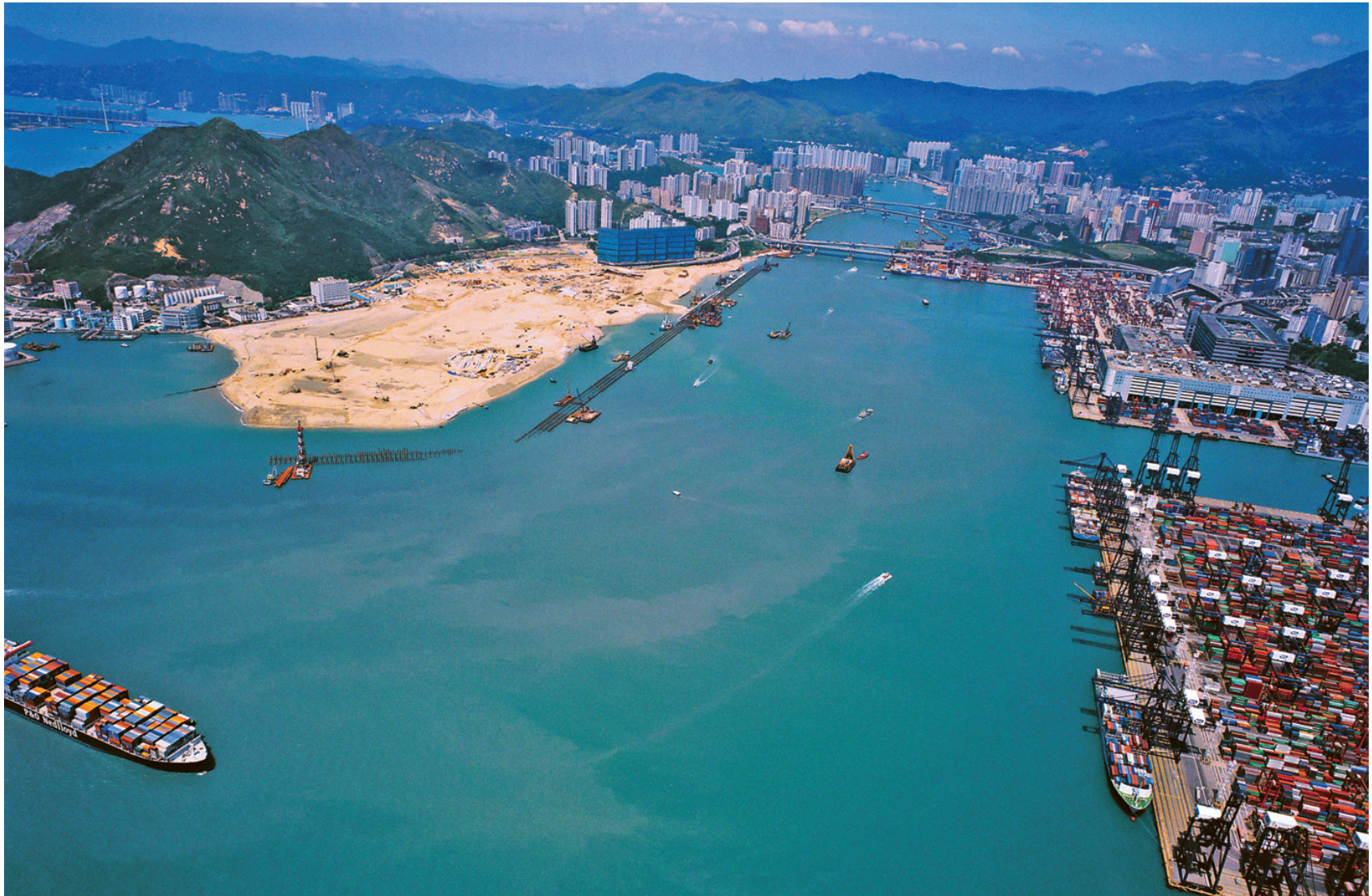
The reclamation and construction of the yard and quay deck of Terminal 9
