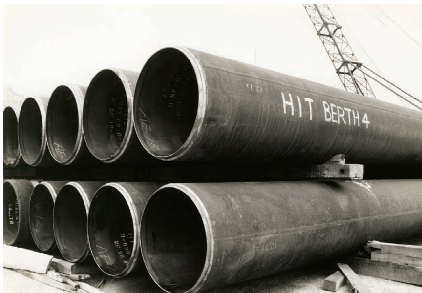
The construction of Terminal 4 involved over 40,000 metres of steel piling, which were driven into place to form an 881-metre-long quay with three berths
