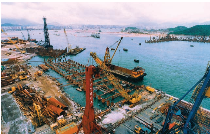
Above: A view of the construction of the two berths and the cross wharf of COSCO-HIT. Terminal 8 East was built adjacent to HIT's terminals
