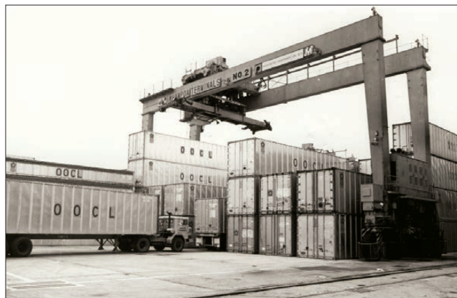
1-over-3 rubber-tyred gantry cranes (RTGCs) were used in the 1970s
