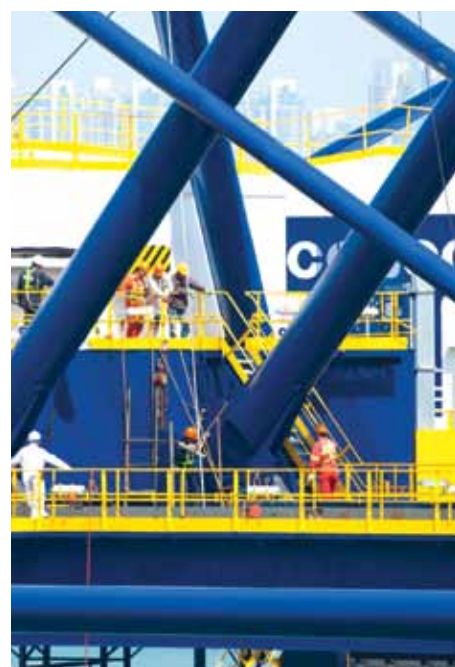
Staff on the upper deck of the quay crane lowering the A-frame
